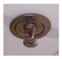
Sprinkler heads should be a set distance apart to make sure that together they cover enough area to put out any fire.
